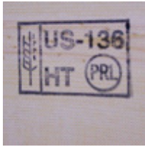
Stamp signifying the lumber used in constructing a crate has been properly treated to prevent introduction of potential foreign insect and fungal pests.
